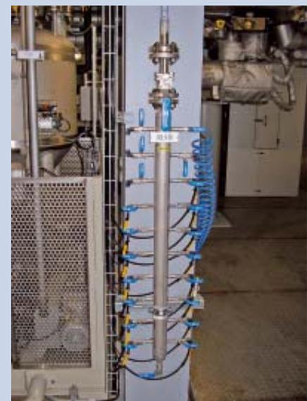
**Manifolds for air-pressure services, manufactured by TEG Germany. RK Proball ball valves for general services, from KLINGER Germany.**
